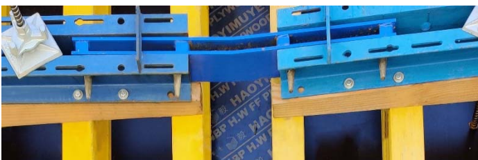
Tie Rod System and Connections Details
