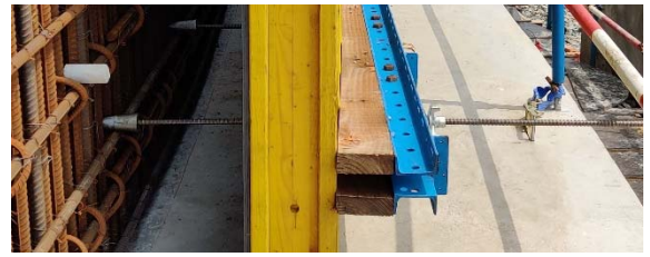
Tie Rod System and Connections Details
