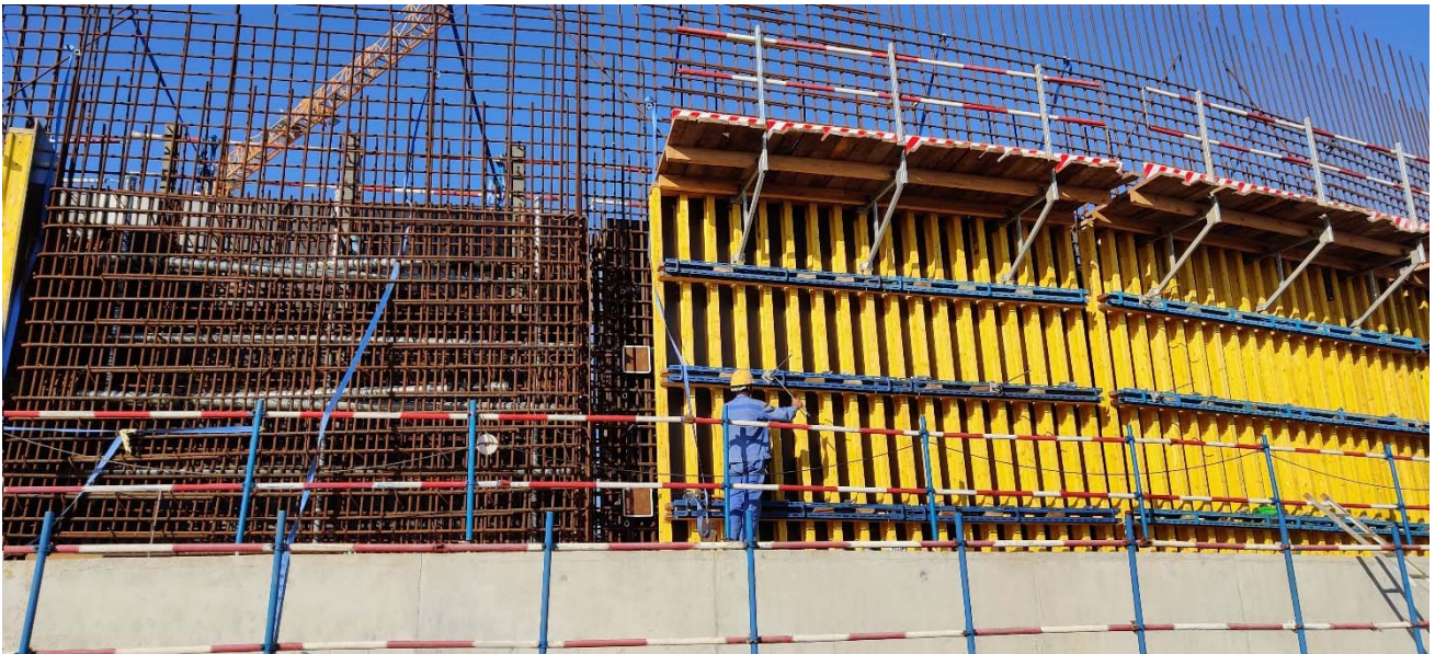
Formwork Unit Installation
