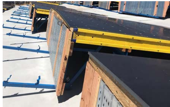
Upper Platform Hanger Assembly Details
